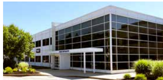
RELYCO's headquarters, Dover, New Hampshire
